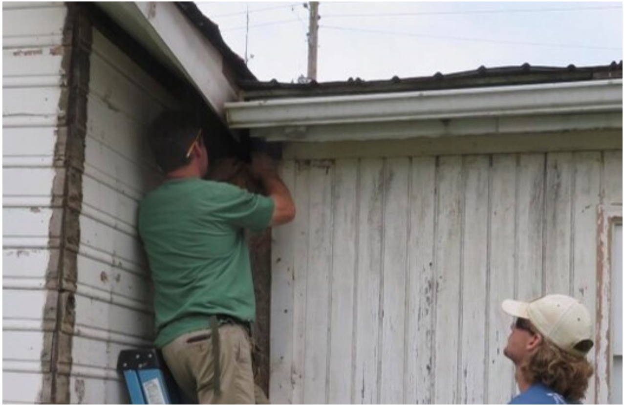
Working on the buildings. © Main Street Middletown, MD Inc.
